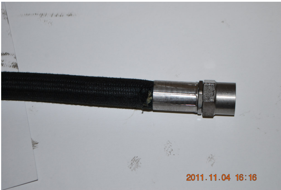
Photo14. Damage to the hydraulic hose of the landing gear extension system of SP-LPC airplane.
